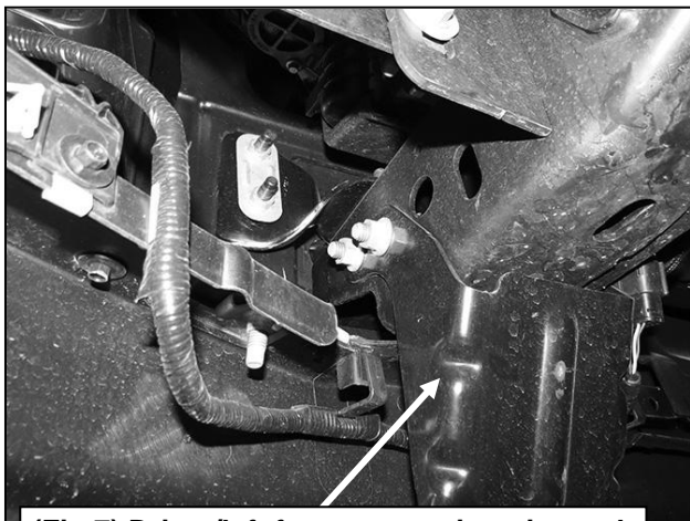
(Fig 7) Driver/left frame extension pictured
