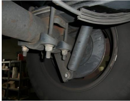
Work on one side at a time to prevent driveline damage. Remove lower shock Bolt
