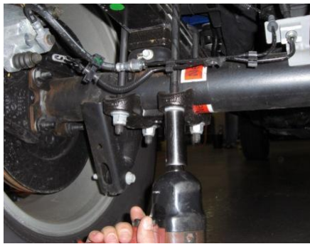
Loosen and remove factory u-bolt hardware.
