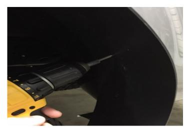
7. Install the SS self drilling screws at the other pre-drilled locations evenly around the flare.
