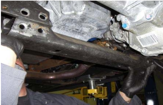
37. Re-install the rear cross member as original.
