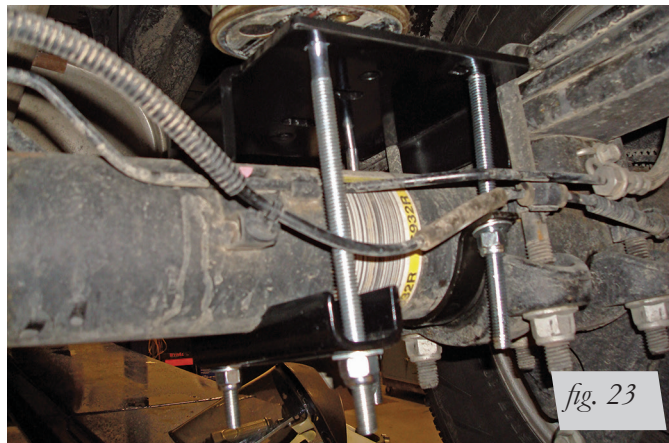
Right side (passenger) view towards rear of finished installation torqued to 10ftlbs.
