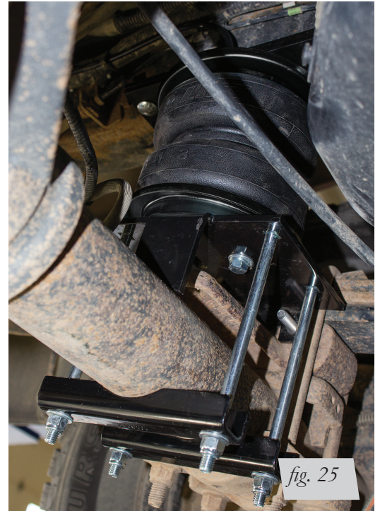
Left side (driver): front view of installation.
