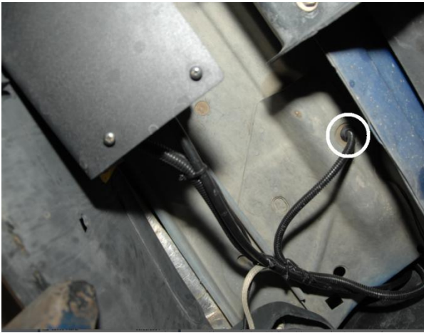
Image K - Location of the two 12-volt wires for switched power (ignition) and your horn button, routed into cab through floor on passenger side.
