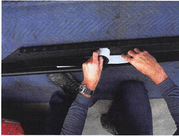
Figure 4: Rolling the tape onto the rails
