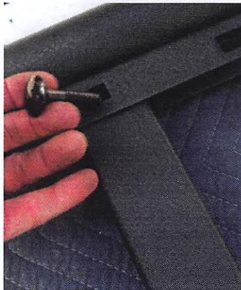
Figure 26: Carriage bolt being installed into racking tube
