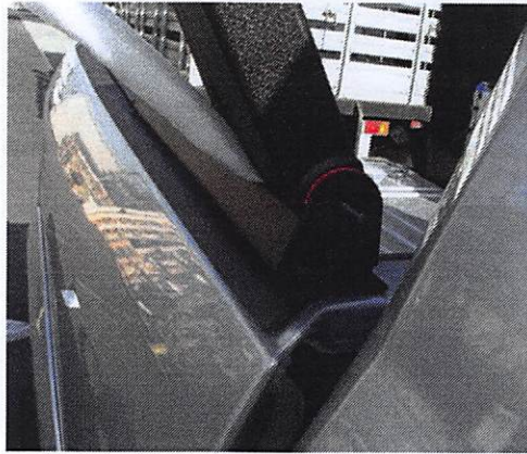
Figure 19: The foam placed in-between the riser and rail for protection.
