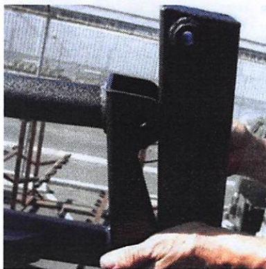
Figure 24: Rack assembly ready to be mounted to the riser assembly
