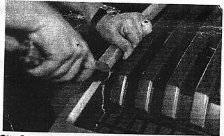
**Step2.** You will need to cut the center portion of the stock grille to allow the new grille to be installed. To cut the center bars you will need any type of disc cutter or saw. We recommend to mark out a 1/4 inch border with a marker to allow you to see where you will need to cut. You may cut the bars right to the edge of the inner leaving it flush to the edge.
