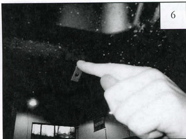
Place Clip (CL1-0011) over existing factory hole.
