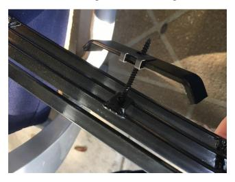
3. Starting with the bottom section, slide the grille overlay into the bottom opening of the grille and tighten screws while holding the brackets in a vertical position. You will need a second screwdriver to hold the brackets in a vertical position while tightening the screws. At this time only tighten screws up just enough to hold the grille in place.
